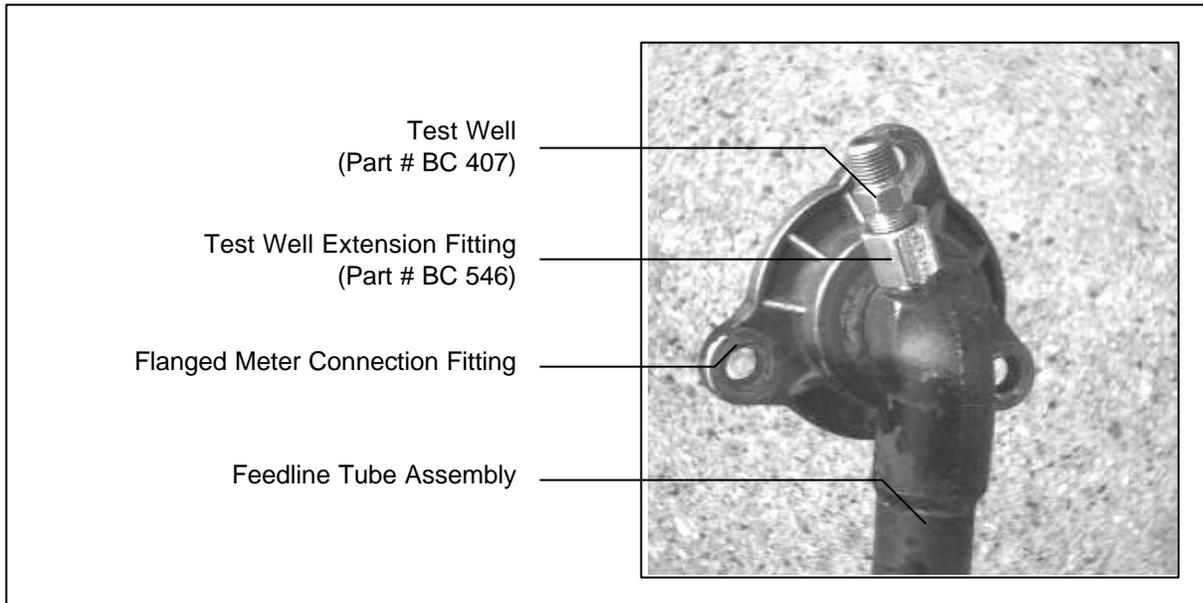
11. Re-connect the feedline tube assemblies, by following steps 3 to 7 in reverse order . (Apply new thread sealing when reattaching the flanged fitting and elbow)
